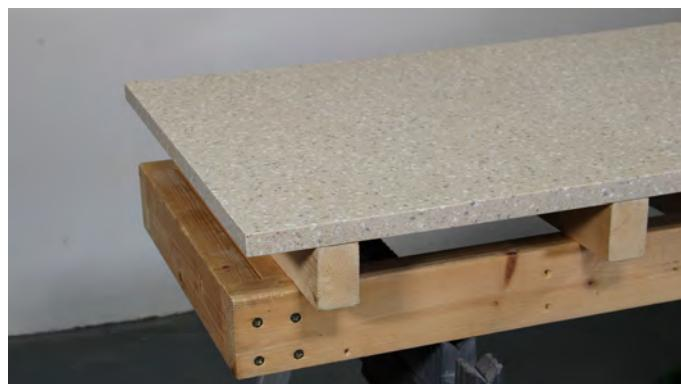
Using the pencil, transfer the dimensions from the plans onto the worktop and mark out where the worktop is to be cut.
