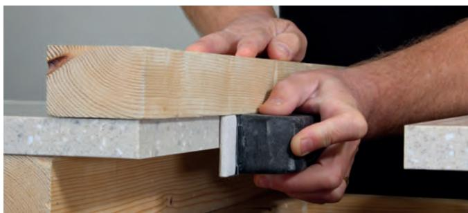
Check there is no print on the underside of the worktop near the edge to be jointed. If so, remove it by sanding with a P240 grit disc as it can contaminate the joint.
