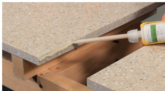
Using the spatula, spread the adhesive so that you have a thin, flat film covering the entire joint face.
