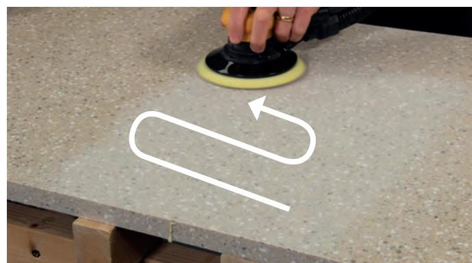
Repeat these processes until the adhesive bead is perfectly flush through the joint and into the worktops.
