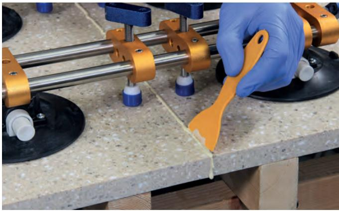
To do this, simply cut a small 45° angle on a piece of 90° card and slowly drag up the internal joint removing the excess adhesive.
