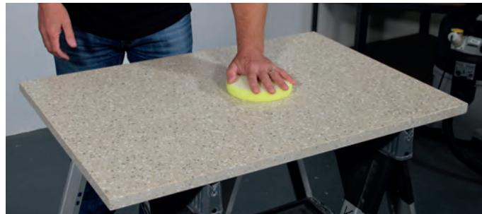
Make sure that all edges and router detailing such as undermount sink cut-outs and drainer grooves receive the same application.
