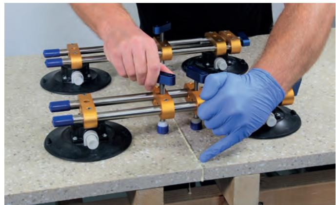
The worktops may have slight variations in thickness due to manufacturing tolerances so all you are doing is evening out the difference in levels to minimise the sanding that will be required.
